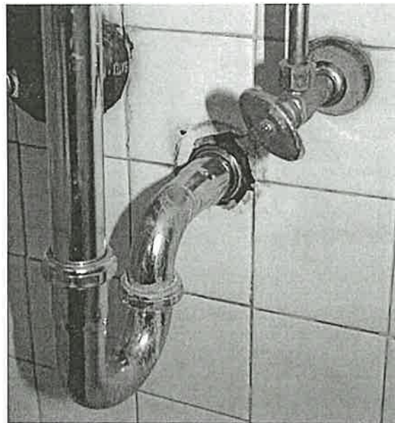
Figure 4-20. Pipe penetrations into the wall need to be sealed to prevent cockroach movement into the area.
