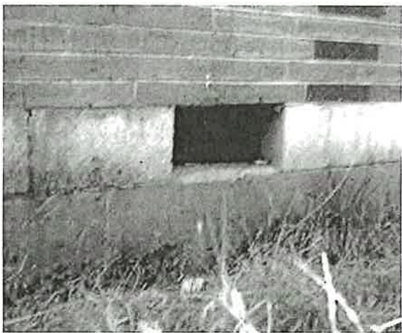
Figure 2-13. Properly screened vents prevent rodents and other pests from gaining access.
