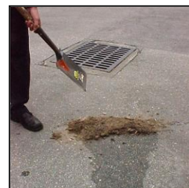
Dirt from close by prevented the spilled material from entering the storm drain
